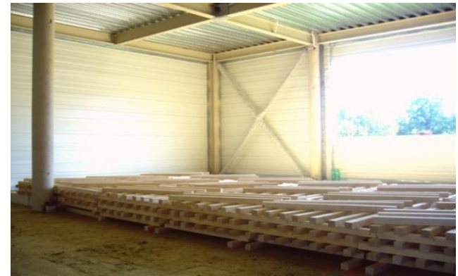
Fire load before the test
